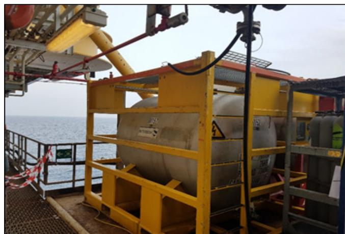
▲ Emptying of line went into a separate tank to start out with a high turbulent flow (high Reynolds number).
