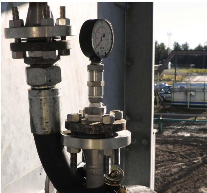
To carry out this cleaning process - called flushing - you use a plant which is successively connected to the hydraulic system at different places until the whole system has been cleaned.
