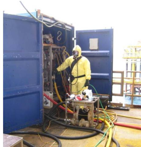
Known and well-tested equipment for the de-scaling procedure is placed on a service vessel.
