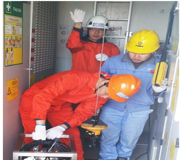
▲ Hoisting in a GE WTG on site
