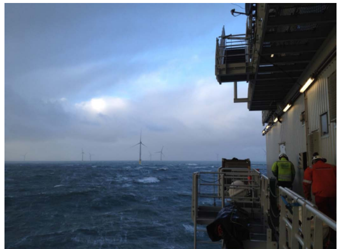
▲ OTW work on a substation
