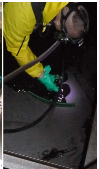
▲ Mechanical cleaning of tank
