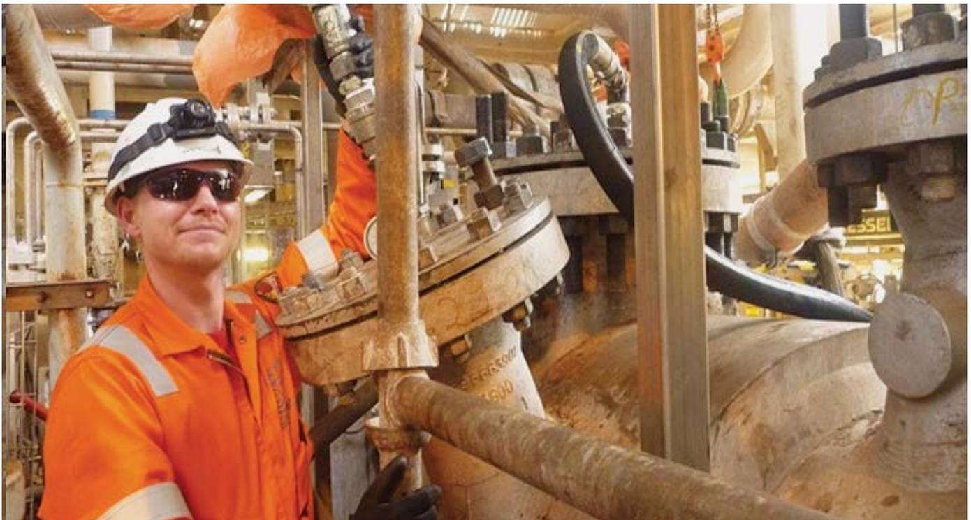
**Picture 2** – Connecting Ocean Team's chemical cleaning unit to the gas compressor. Efficient and quick cleaning without dismantling, shipping and disassembly of the compressors. The results were large savings in time and money.
