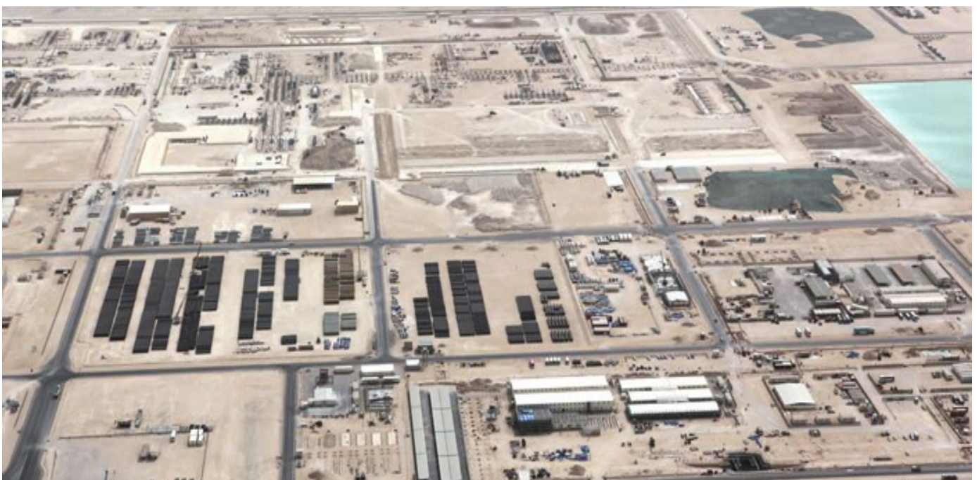
Aerial View – Barzan Onshore Plant ▲
