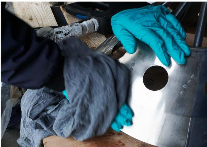
▲ *Last part of the process - drying off thin film.*
