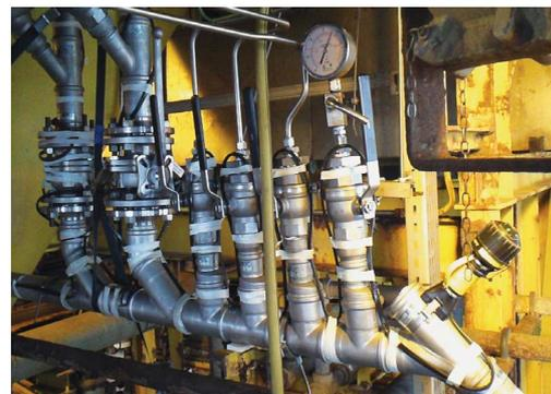
◀ The newly installed pipe system. In order to avoid frost skips, they dressed the pipes in heating cables.
