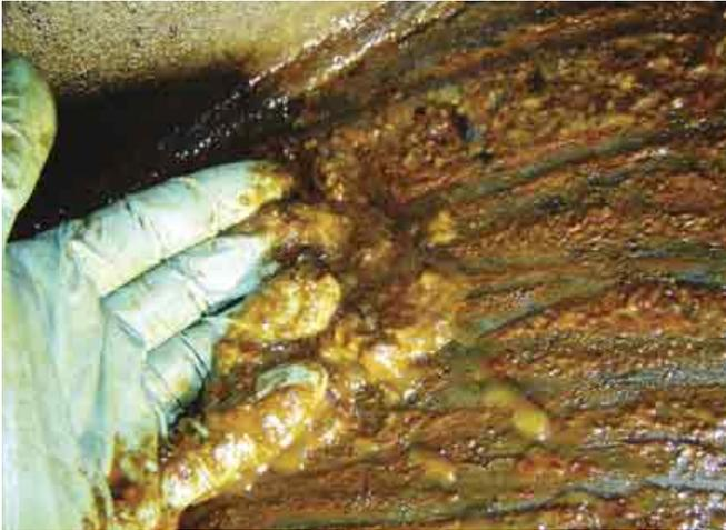
Picture 3 - Sludge on reservoir.
